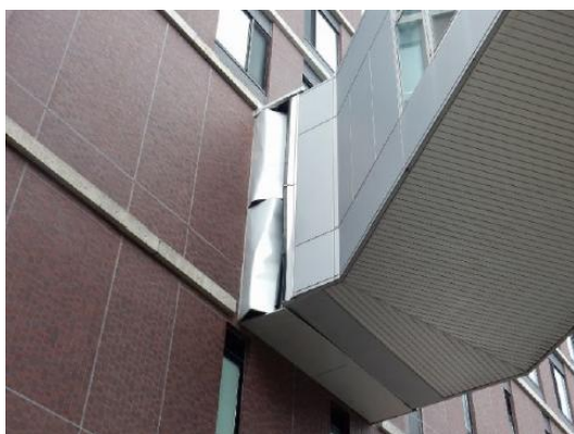
Photo 4: Damage to the SI Exp. J panel
