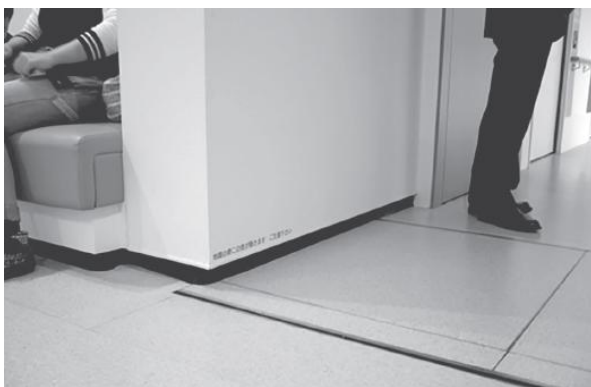
Photo 5: Exp.J and sleeve wall between the seismically isolated building and the seismic resistant building
