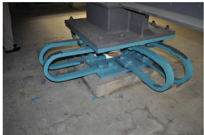
Steel damper after the quake
